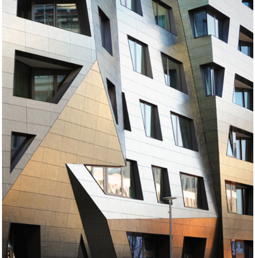
The Sapphire apartment building in Berlin is coated in a layer of titanium dioxide that allows the facade to clean itself, and the air around it, when exposed to natural light. Photo: Thomas Kolbein Bjørk Olsen
